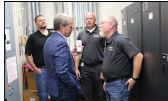
Governor Pilleen discusses the operation and construction of the back up generator switch gear with maintenance manager, Mike Heaps. This is part of the State's information technology infrastructure.
