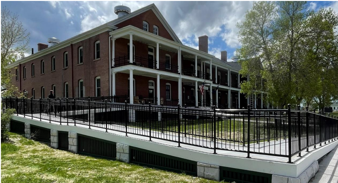
Nebraska's Fort Robinson Lodge after an ADA ramp upgrade.
