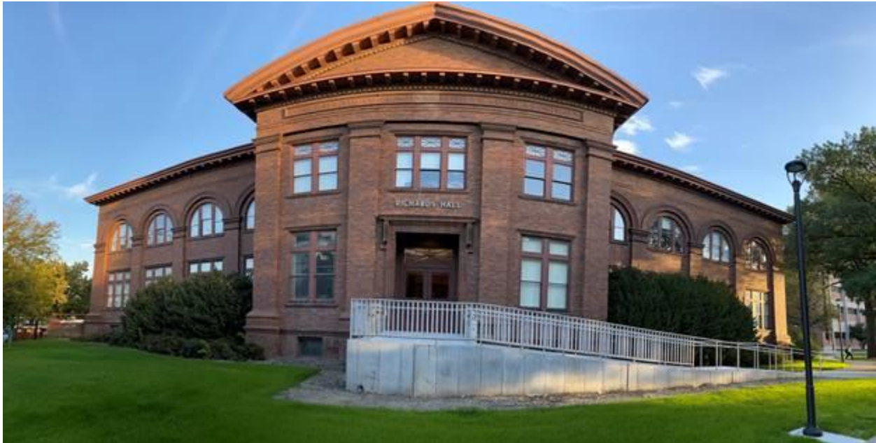
University of Nebraska-Lincoln's Richards Hall after ADA accessibility upgrades.
